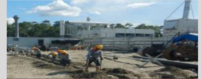
Workers are trained and certified so they may get good paying jobs in the future
