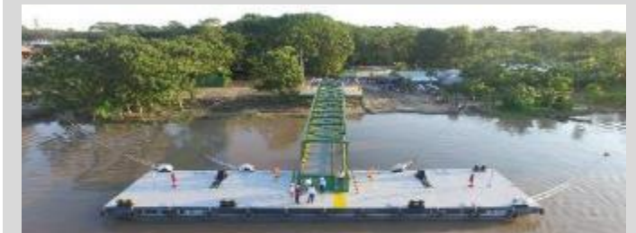
$0.5 million Bretaña dock built by PetroTal will help empower the Bretaña municipality
